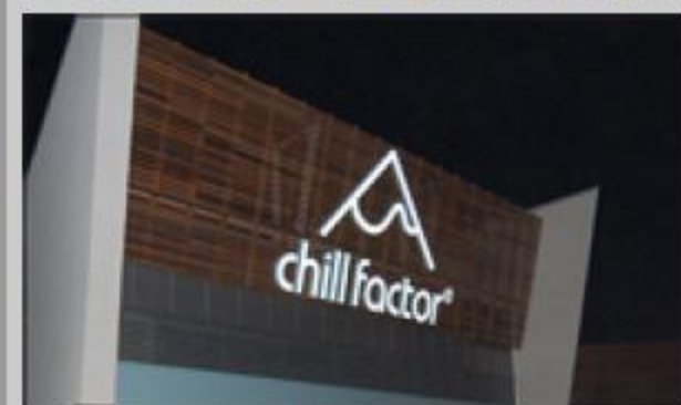
Chill Factor, Manchester Fire Detection, Voice Alarm/Public Address, Intruder Alarm, CCTV, Access Control, Intercom Systems, Disabled Refuge
