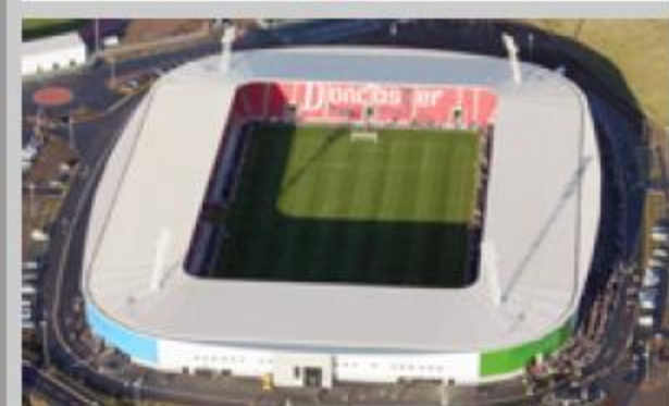
Doncaster Keepmoat Stadium - Doncaster Design, Supply & Installation of Fire Alarm, VEPA & Air Sampling
