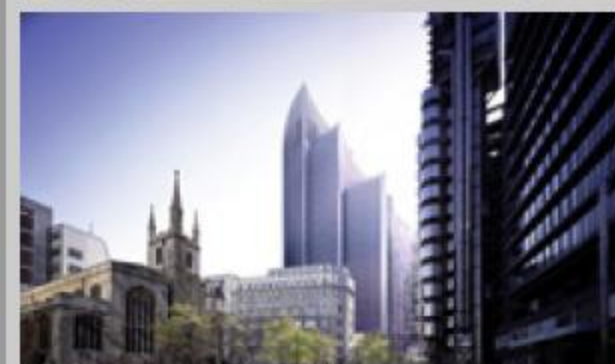
The Willis Building, 51 Lime Street - London Design, Supply & Installation of Fire Alarm, VEPA, Emergency Voice Communication, Disabled Toilet, Aspirating Fire Detection, Water Mist Extinguishing Systems and Roof Vent Controls
