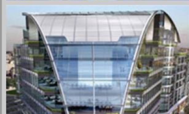
Cardinal Place, London Fire Detection, Voice Alarm/Public Address, Fire Telephones, Disabled Refuge and Graphics
