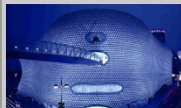
The Bullring, Birmingham Fire Detection, Voice Alarm/Public Address, Fire Telephones, Disabled Refuge, Security, Access Control, Graphics, Extinguishers
