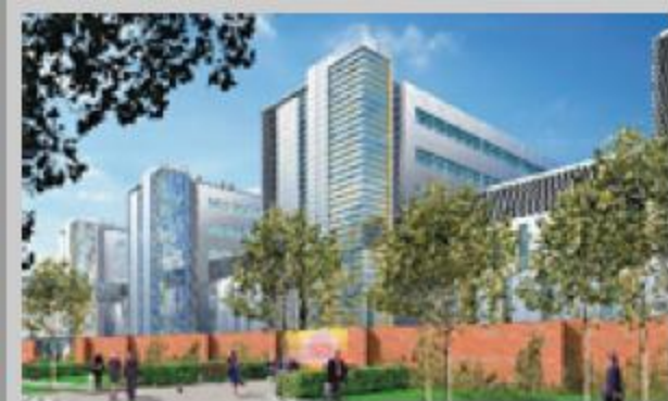
Manchester Royal Infirmary - Manchester Design, Supply & Installation of Fire Alarm and Integrated Smoke Damper
